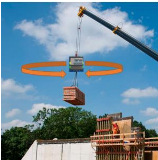
Figure 1- Online monitoring of all lifts and Roborigger performance and productivity
