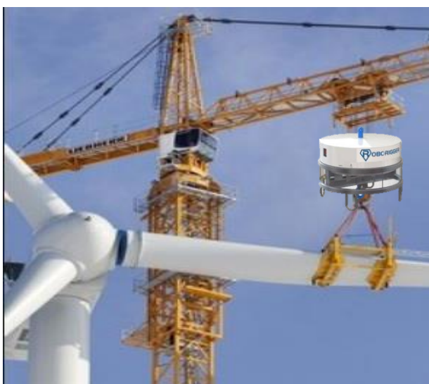
Installing wind turbine blades
